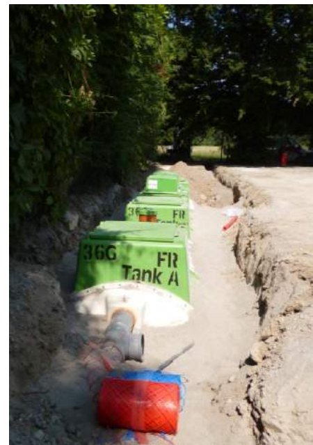
Micro-station Tricel Novo FR36 installée
